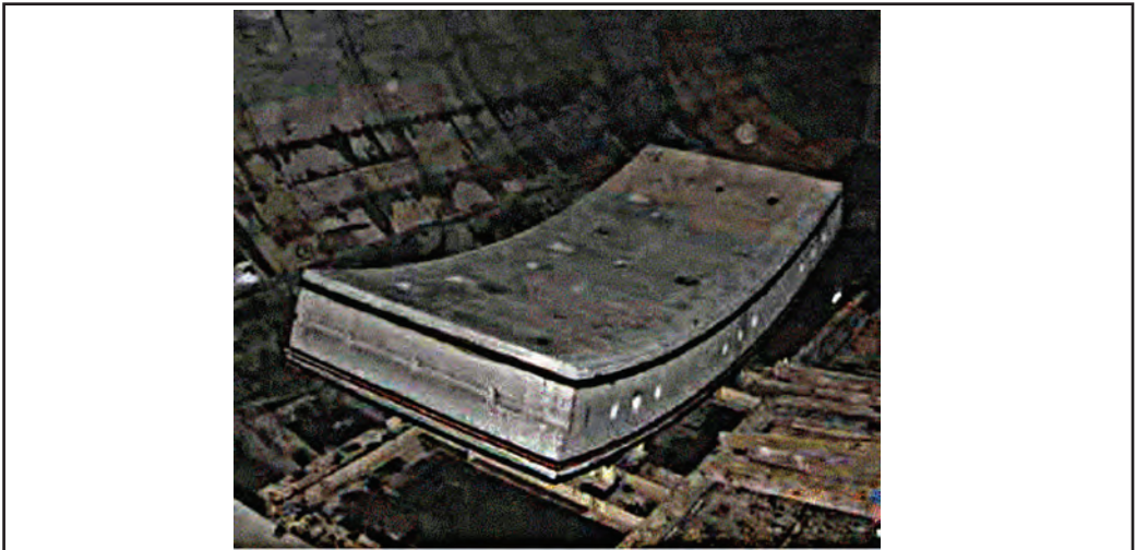
Figure 21. Precast Concrete Segment with Double Gasket (EPDM and Hydrophilic)
