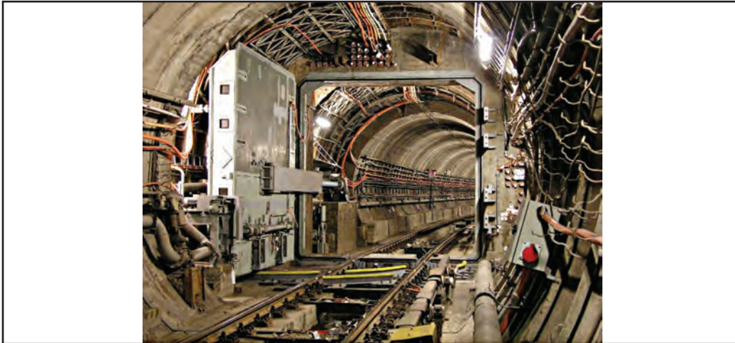
Figure 24. Hydraulically Operated Hinged Floodgate
