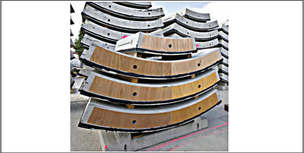
Figure 20. Precast Concrete Segment with EPDM Gasket and Wood Compression Packing
