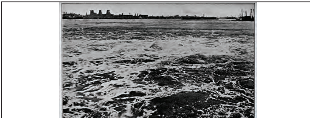
Figure 11. Photograph of a "Blow" During Construction, as Seen from the Surface
